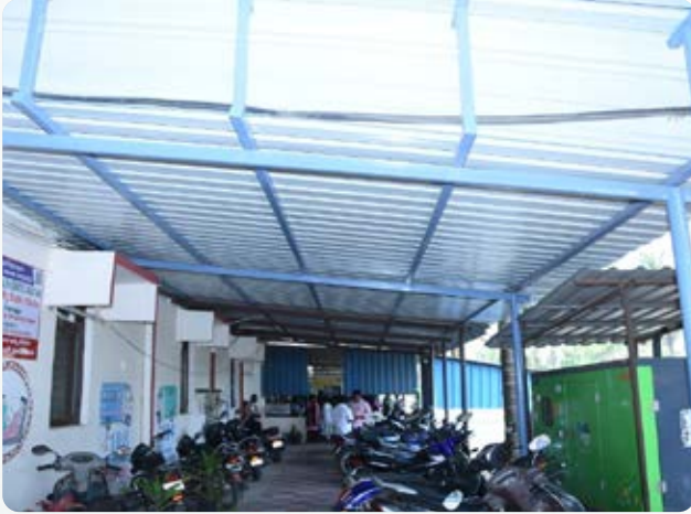
Parking Entrance Shed
