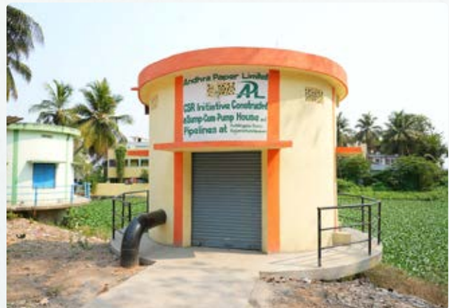
Constructed sump cum pump house and main water line at kotilingalapeta, RJY to prevent flooding in rainy season.
