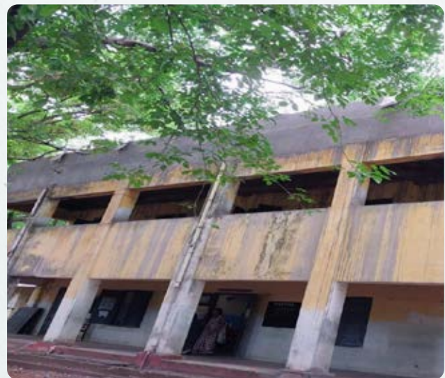
Construction of roofshed to main building at SKVT High School, Danvaipeta, Rajahmundry
