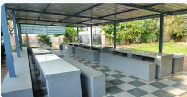
Infra support (Construction of Boundary wall, Dining Hall and Toilets) to 5 MPP Schools in Kadiam Mandal.
