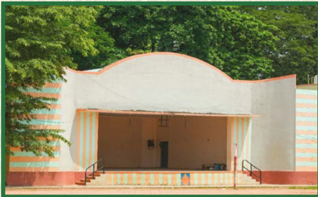
Renovation of Auditorium at APPM High School, Rajahmundry
