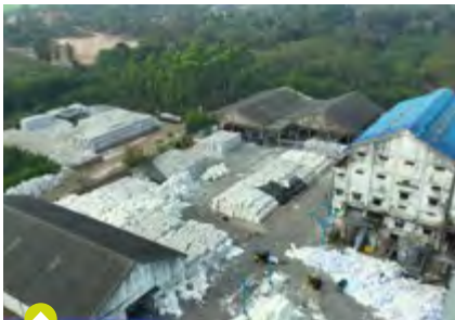
Waste Paper recycling plant
