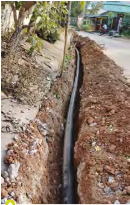
Laid pipelines in Kadiyam Village
